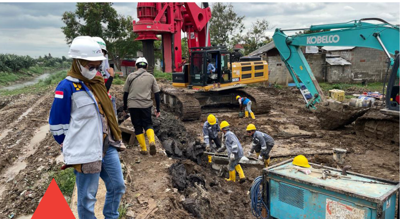
Nona Ritayanti supervising construction of new roads and drains in Makassar.
